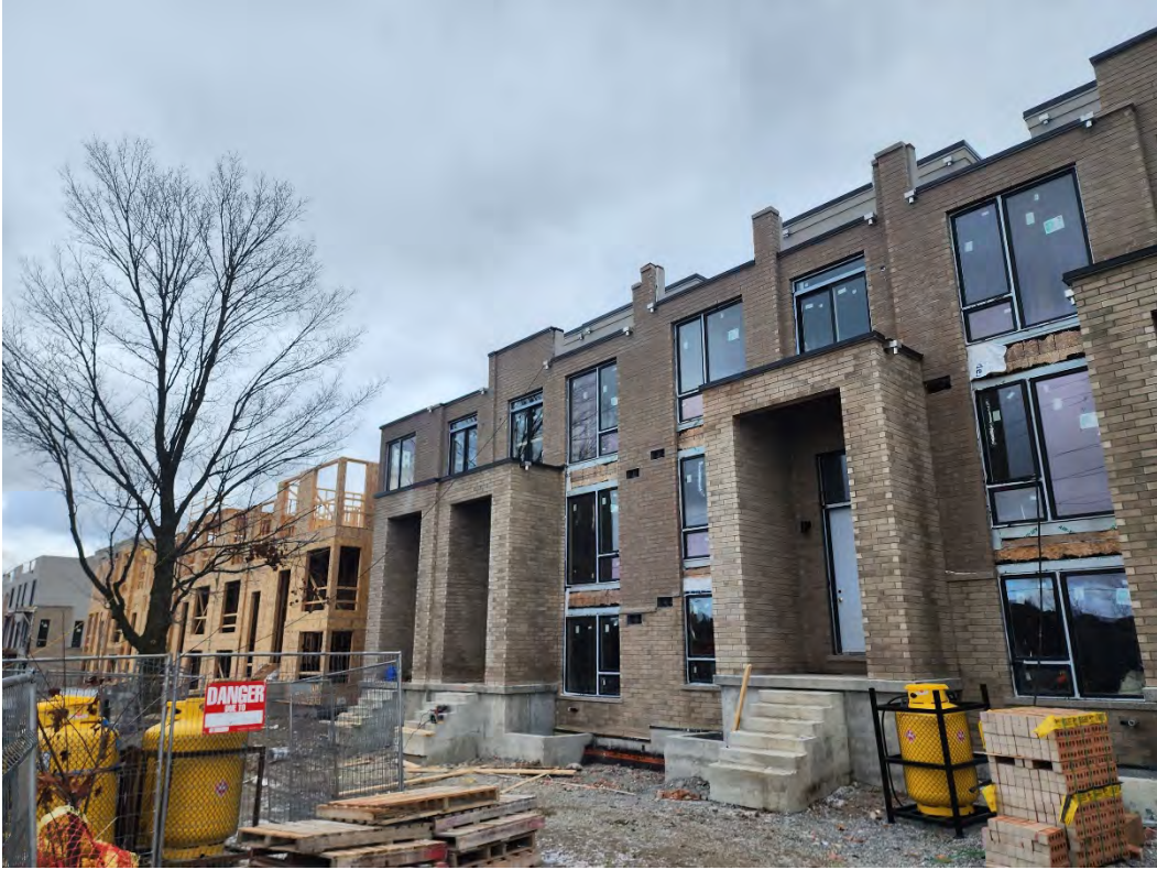
Site Inspection – Block A - December 11, 2023
