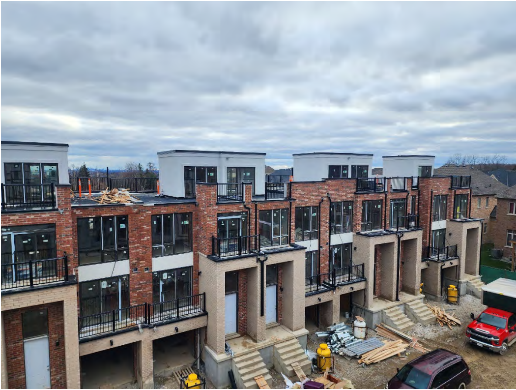
Site Inspection – Block E - December 11, 2023
