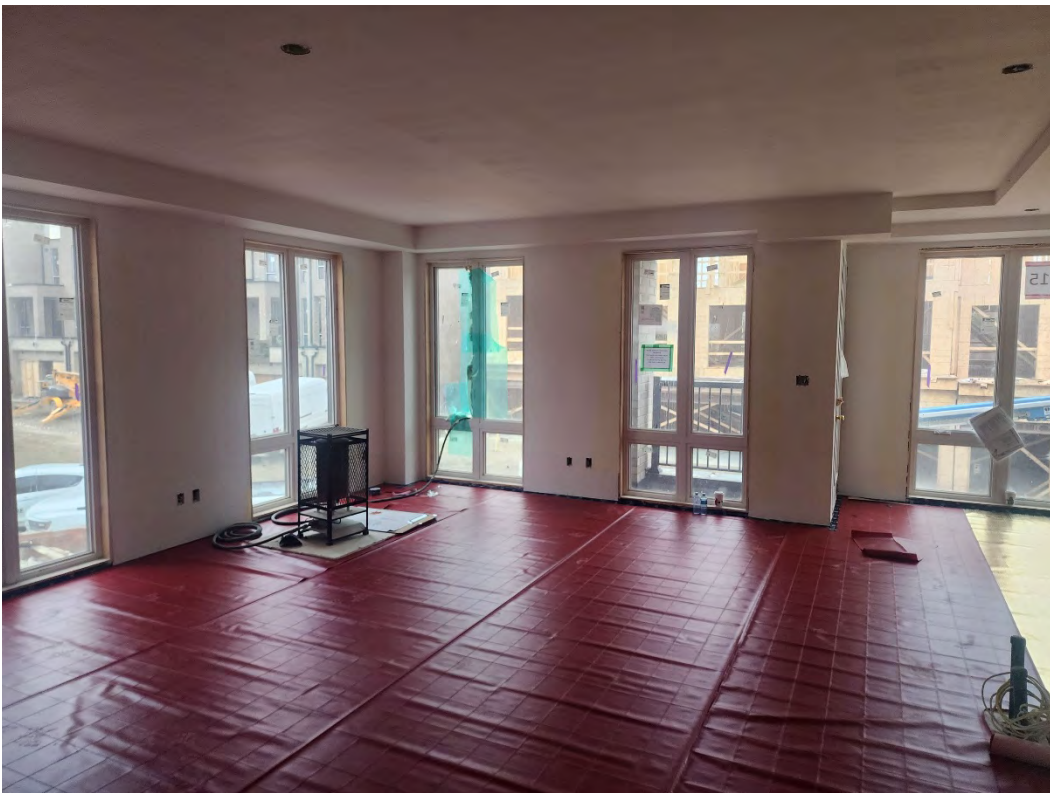
Site Inspection – Block D - December 11, 2023
