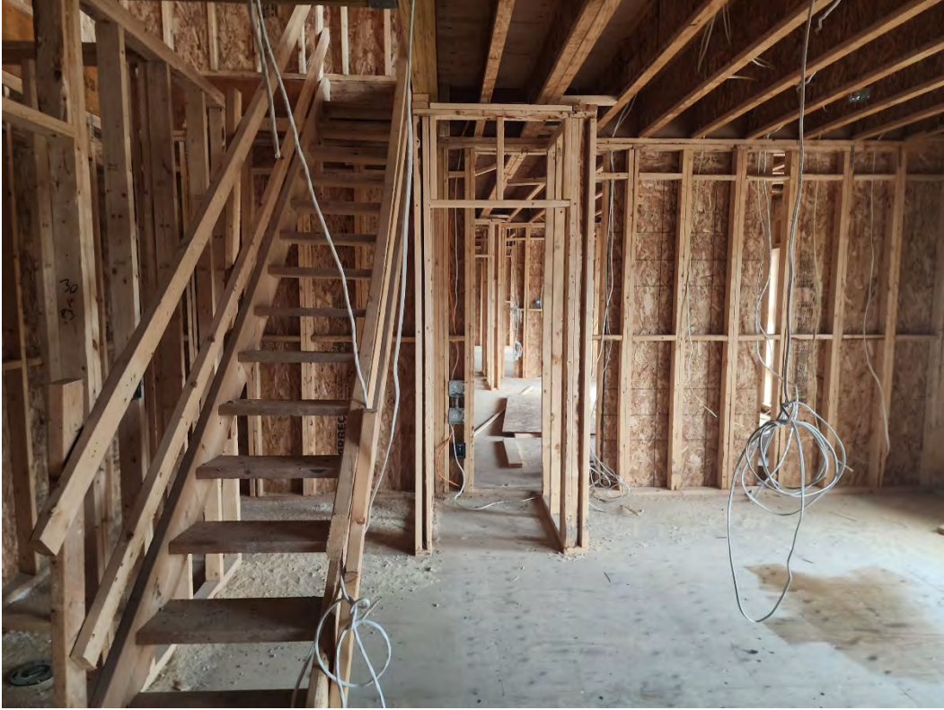
Site Inspection – Block I – December 11, 2023
