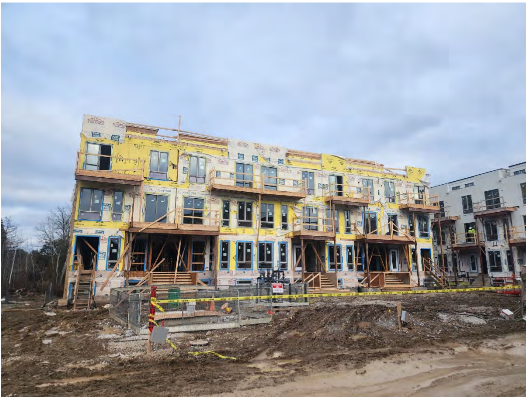
Site Inspection – Block H - December 11, 2023
