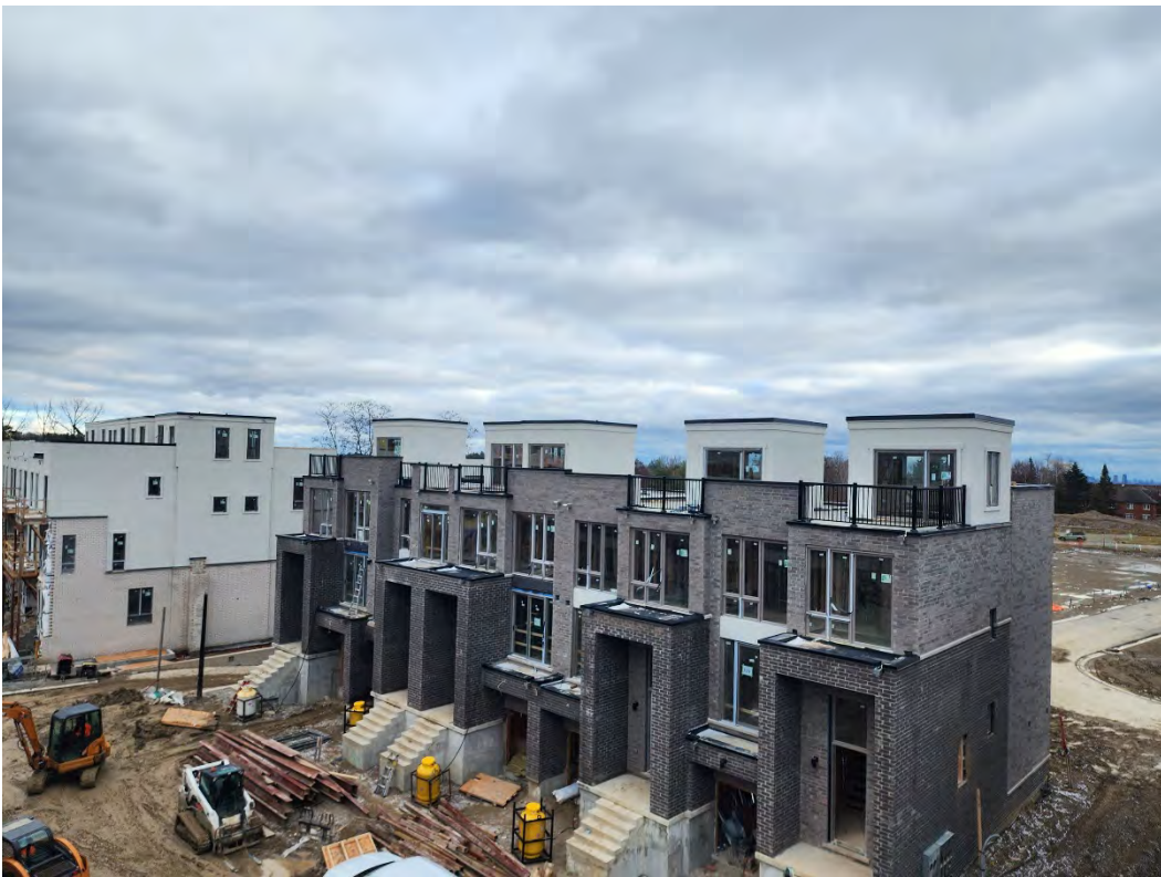
Site Inspection – Block F - December 11, 2023
