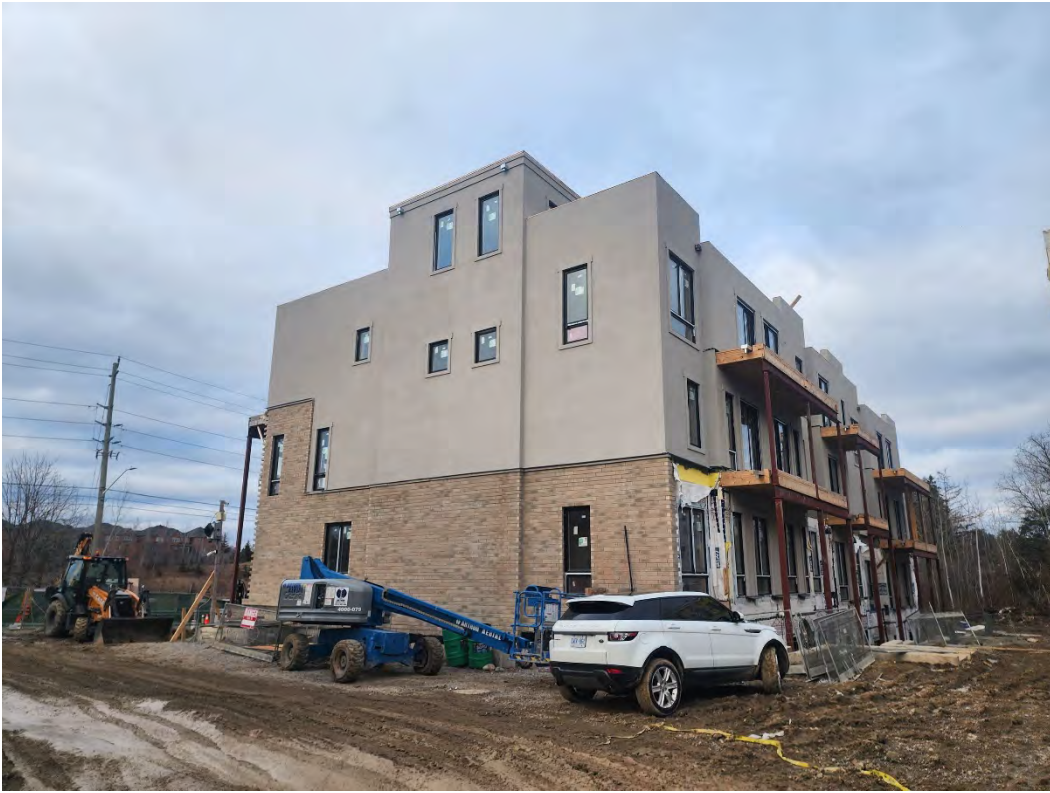
Site Inspection – Block G - December 11, 2023
