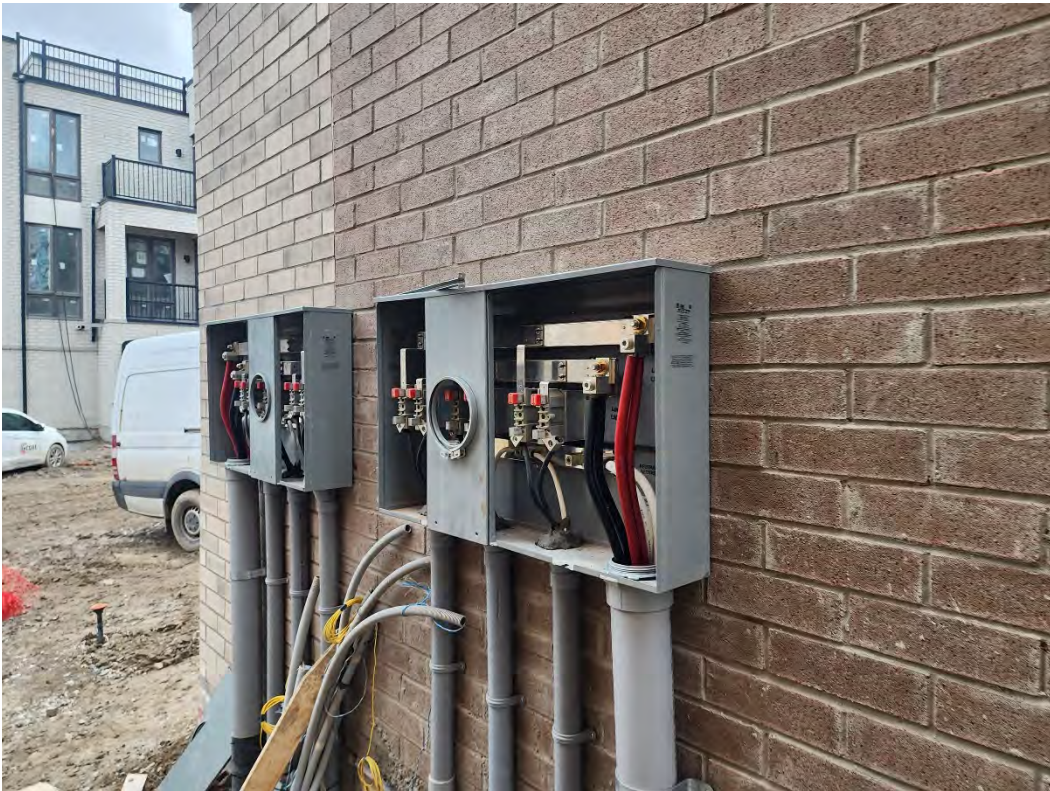
Site Inspection December 11, 2023
