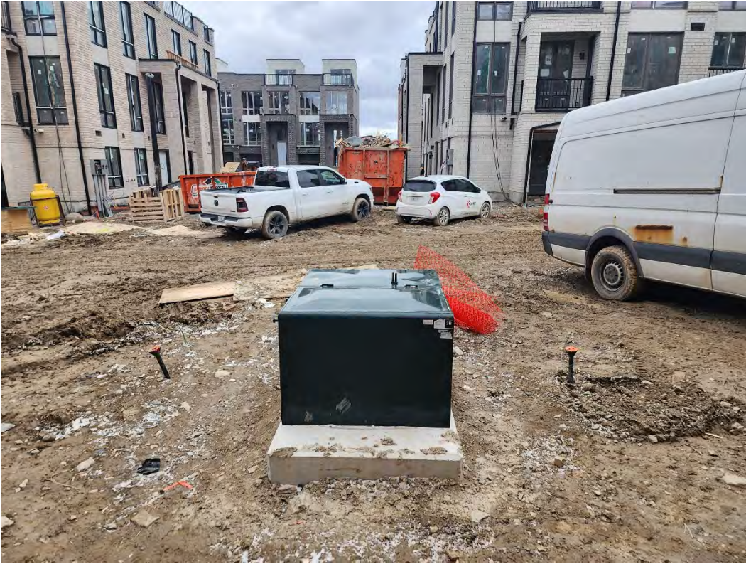
Site Inspection December 11, 2023
