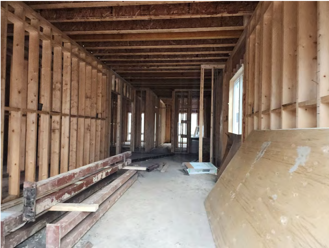
Site Inspection – Block H - December 11, 2023
