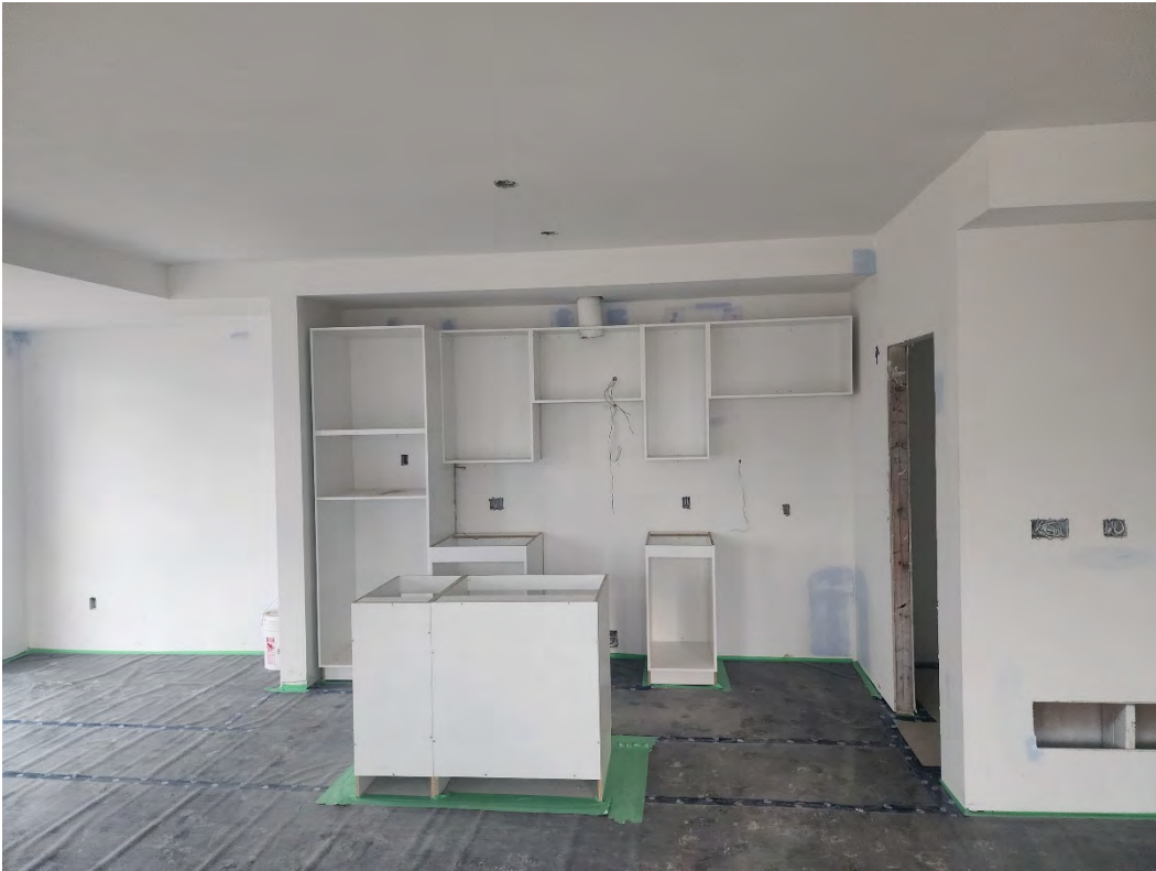
Site Inspection – Block C – December 11, 2023
