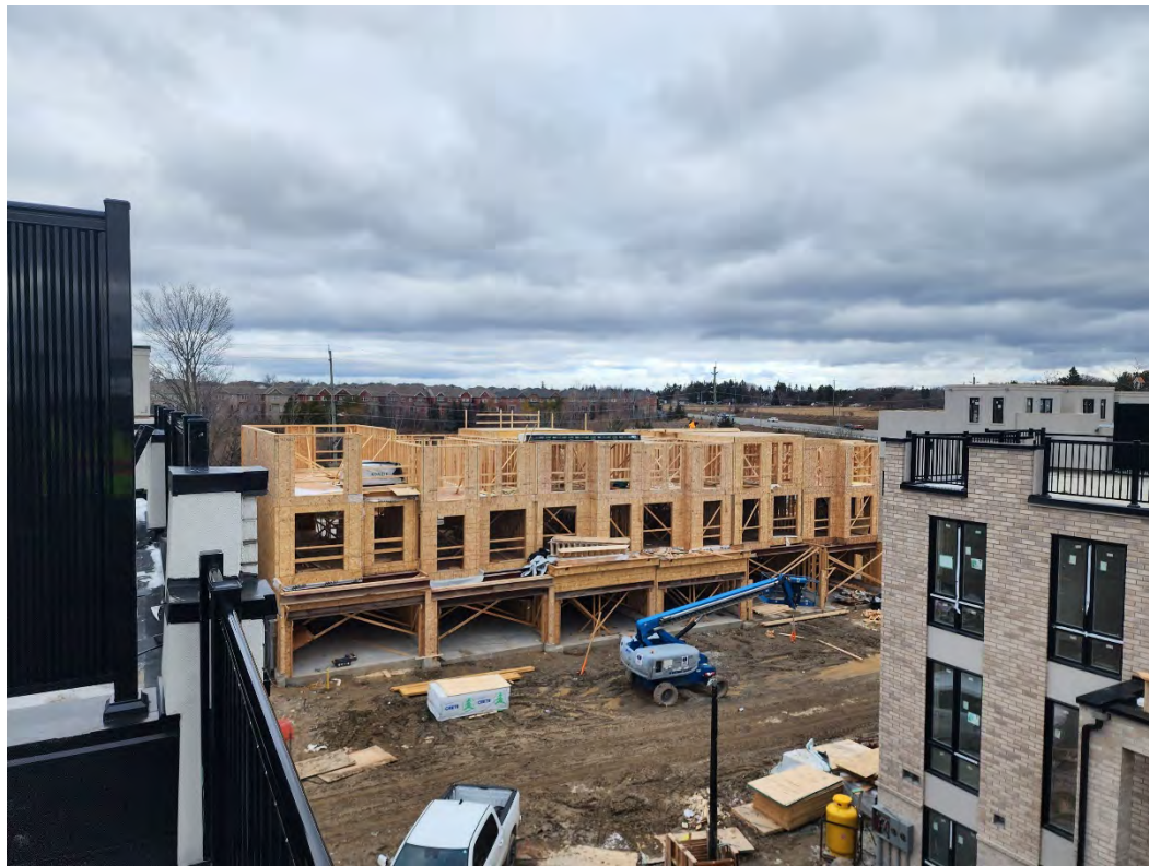
Site Inspection – Block B - December 11, 2023
